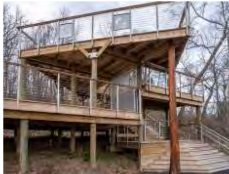
Neabsco Creek Boardwalk, Woodbridge, Virginia
